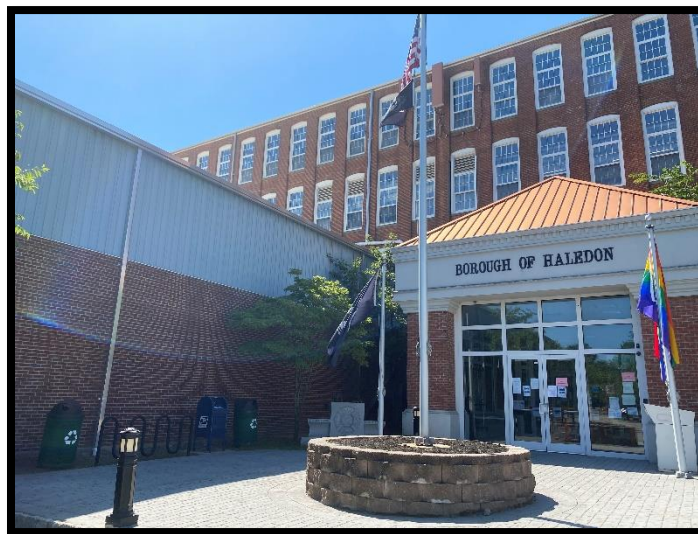
Figure 7 The Borough of Haledon’s Municipal Complex
